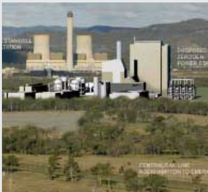
ZeroGen is the 1st power plant in the world to combine IGC and CCS.
