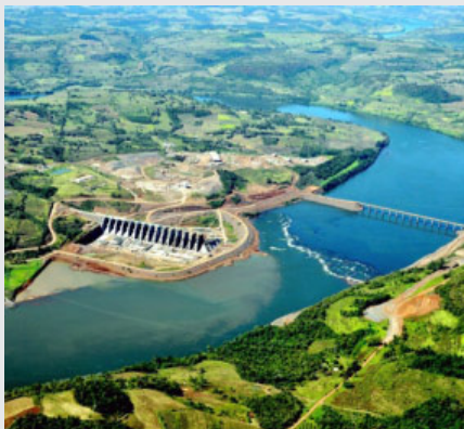
This 855 MW plant now has an innovative tunnel aqueduct and intermediary reservoir.
