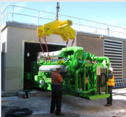
WorleyParsons installed Sewage Gas Engines for wastewater systems.
