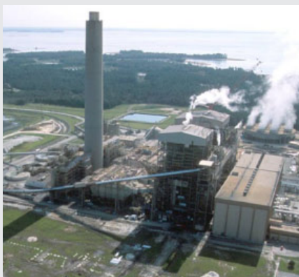
Our creative, overlapping construction plans resulted in saved cost and time.
