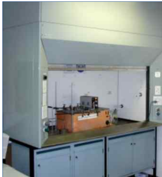
Constaflow fume cupboard.
