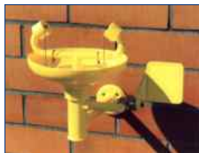
Emergency Eye Wash
